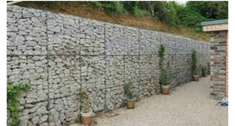
Gabion Basket Retention
